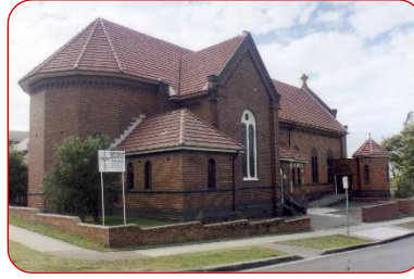
Corpus Christi Church Platt Street Waratah Est. 1917
