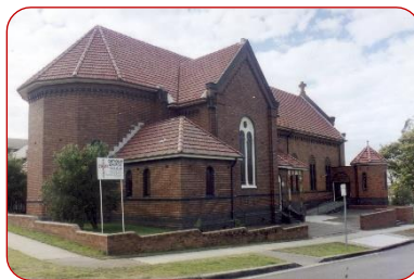
Corpus Christi Church Platt Street Waratah Est. 1917
