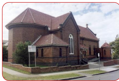
Corpus Christi Church Platt Street Waratah Est. 1917
