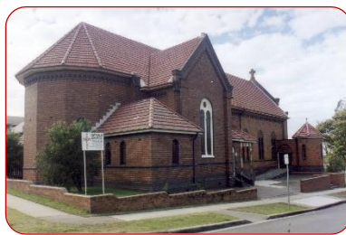
Corpus Christi Church Platt Street Waratah Est. 1917
