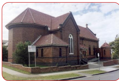
Corpus Christi Church Platt Street Waratah Est. 1917
