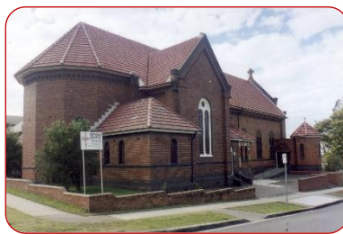
Corpus Christi Church Platt Street Waratah Est. 1917
