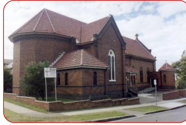
Corpus Christi Church Platt Street Waratah Est. 1917
